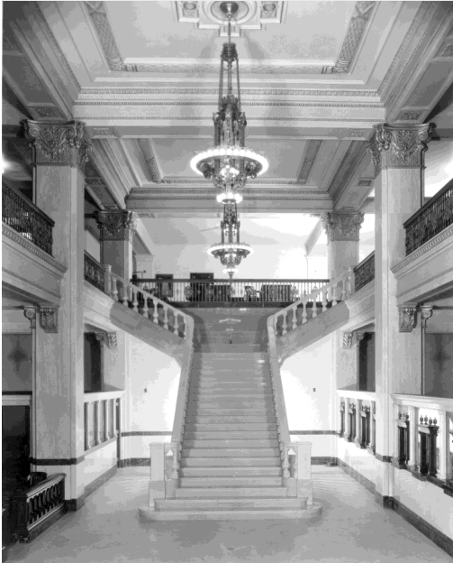
Original Niels Esperson two-story Main Lobby housed The Guardian Trust Company (bank) with a grand staircase to the second level.
